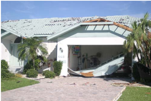
This building survived internal pressurization resulting from the garage door failing. The skin used in these non hurricane rated doors are vulnerable to wind borne debris impacts.
