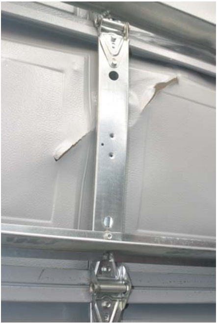
This building survived internal pressurization resulting from the garage door failing. The skin used in these non hurricane rated doors are vulnerable to wind borne debris impacts.
